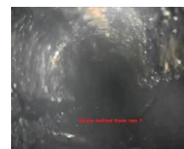
Subsequent camera run post PrecisionCollector cleanout, showing bridge removed.
